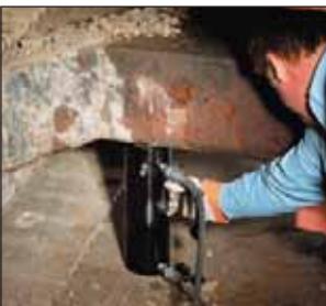
◀ An RAR-506 was easy to position under a bulldozer for repair of frame member.
